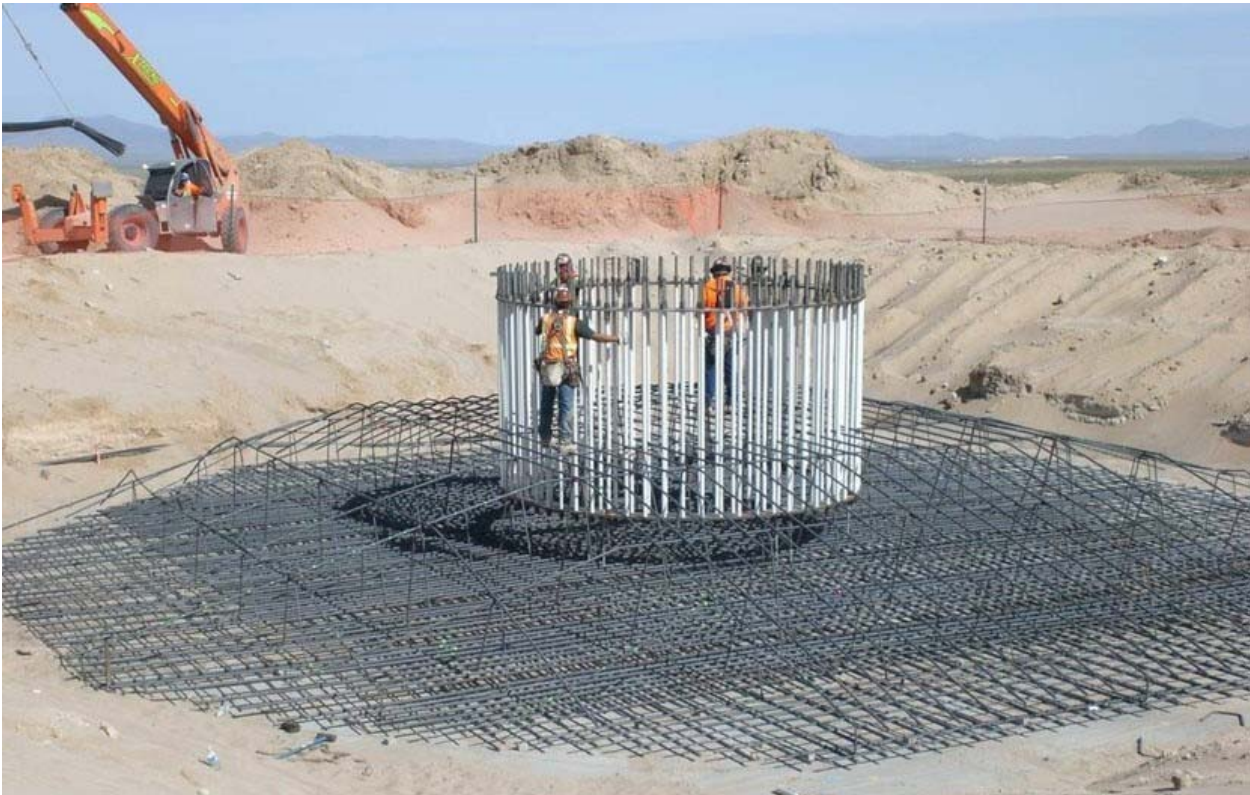
Each wind tower requires a steel rebar and concrete base approximately 50 ft in diameter 8 feet belowground. (Source: U.S. Bureau of Land Management, public domain image.)
