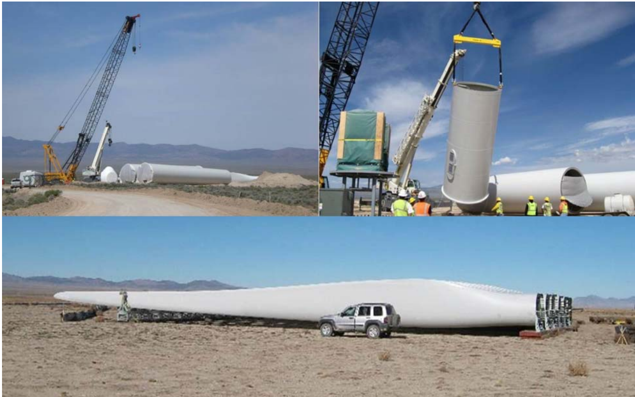
Installation of a typical wind turbine. (Original image source: U.S. Bureau of Land Management, public domain images.)
