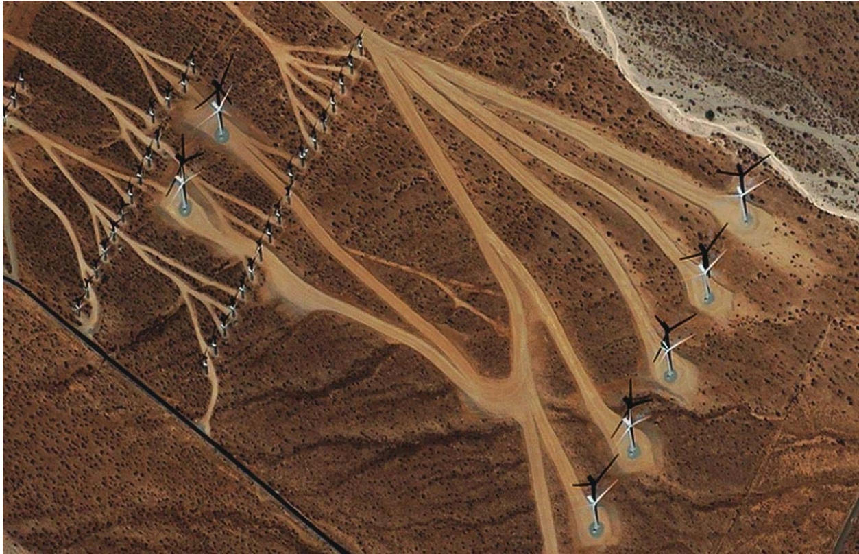
Installing the towers requires access roads during construction and right-of-way for buried cables and maintenance access. (Source: NASA, public domain image.)
