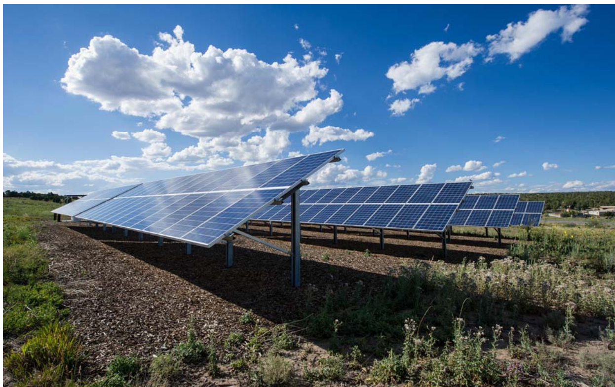
Ground solar photovoltaic array. (Source: National Renewable Energy Laboratory, Dennis Schroeder; image used as permitted.)
