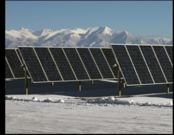
Ground solar energy
