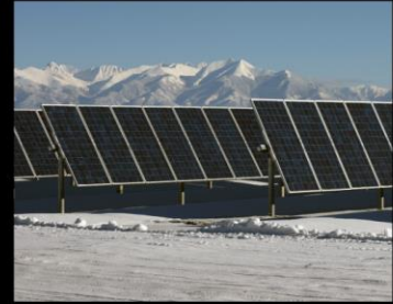
Ground solar energy
