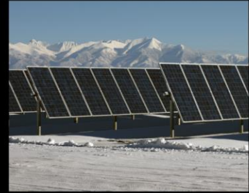
Ground solar energy
